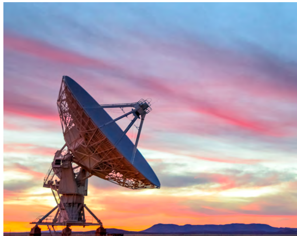
Ground station antenna for gateway
